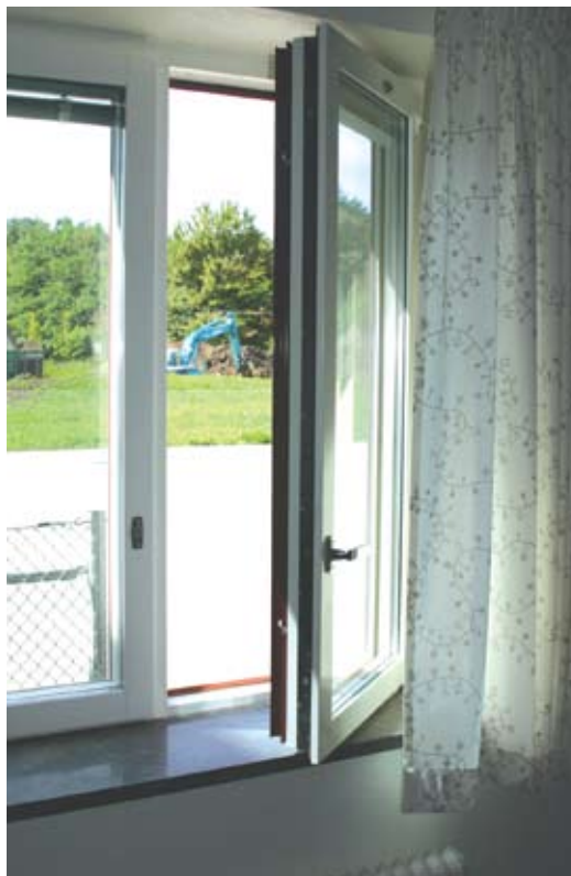
Security system window-contacts are co-utilized by the climate system
